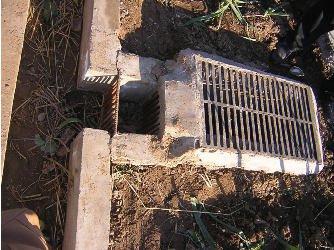
Appendix B.4 The cover of the sediment tank, which is connected with the ditch (studied in Chapters 4, 5 and 6)
