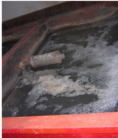
Appendix A.2 Oxygen tank at the Qingzhiyuan plant (studied in Chapter 2) Source: taken by author
