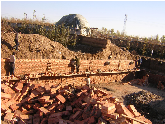
Appendix B.3 Storage tank under construction (studied in Chapters 4, 5 and 6)
