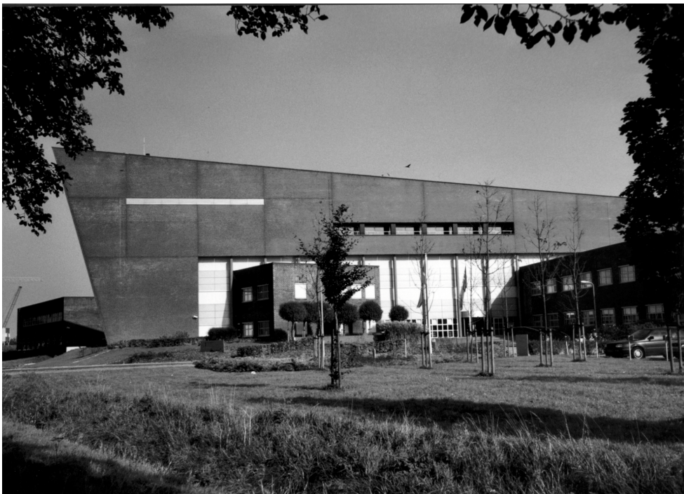
PWN building at Velsbroek
