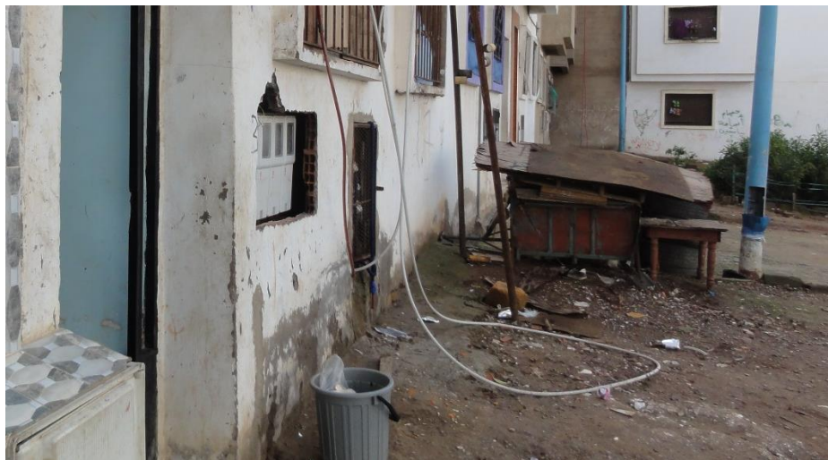
Figure 6-18: Informal connections to the power grid in Nouvelle Lahraouiyyine. Author's picture, January 2017.
