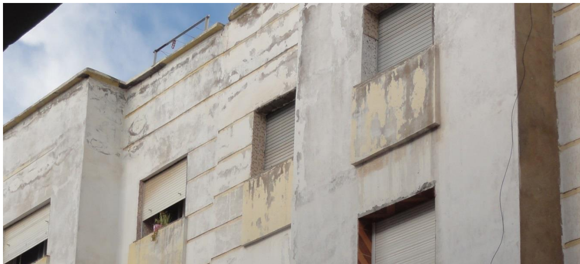
Figure 6-9: Visible damage outside a six-year-old house in Nouvelle Lahraouiine. Author's picture, January 2017.
