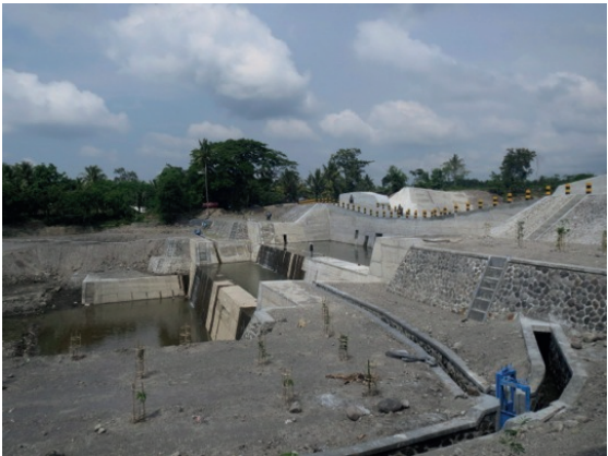
Figure 7.6 Sabo dam as a form of water and lahar management (BBWS SO, 2015)
