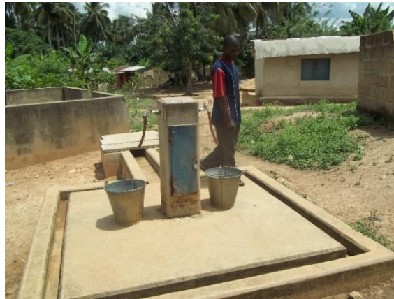
Photo 6.1 Public standpipe with bucket used for measuring water and hose to control the flow of water
