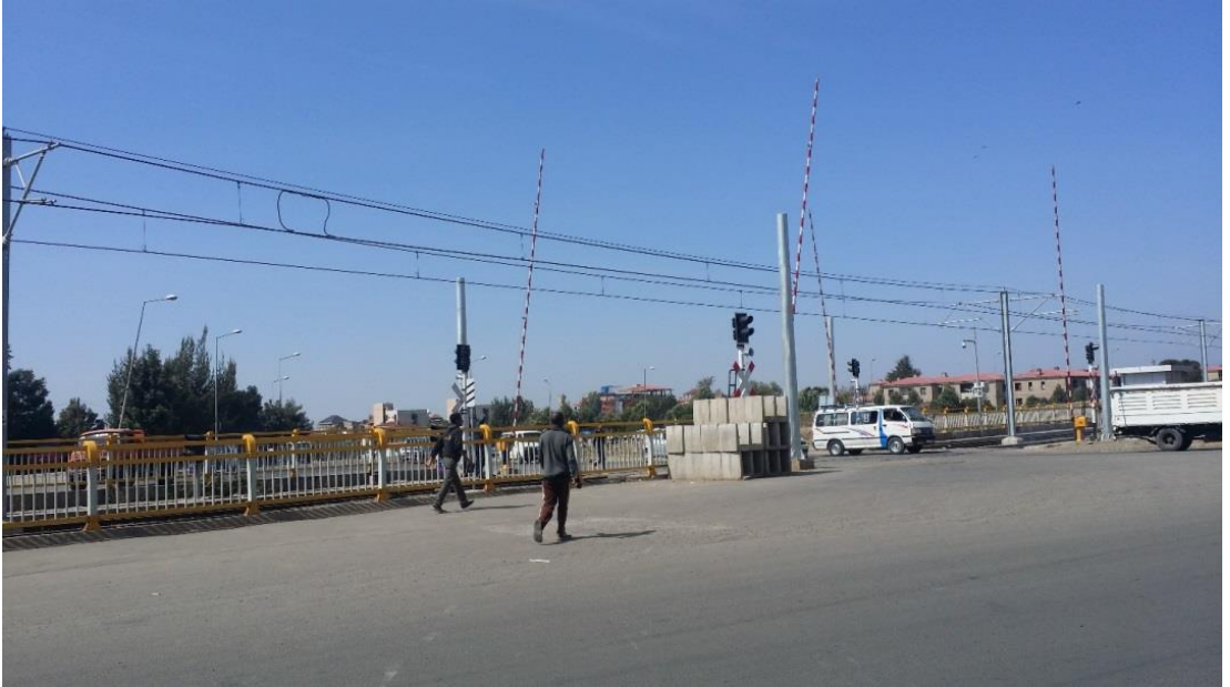
Photograph 9: Intersections constructed and opened-up, with red and white colours bars, for the passage of vehicles at U-turns.
