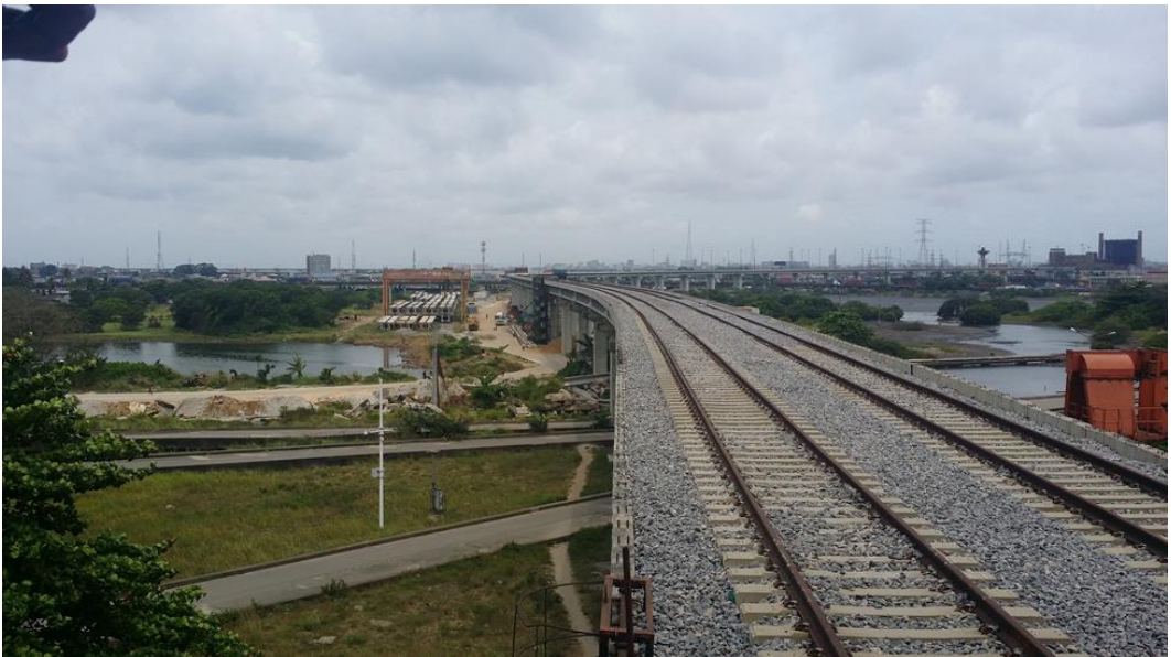
Photograph 12 above shows some of the constructed infrastructures to carry the LRT as a bridge, with roads and waterways beneath it, along the national theatre route in Lagos city.
