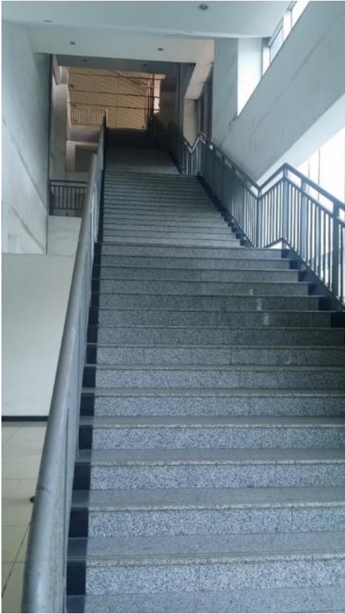
Photograph 22: Staircase at National theatre station Lagos LRT
