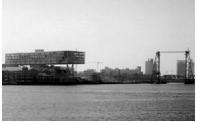
The new Unilever building &amp; the old railway bridge
