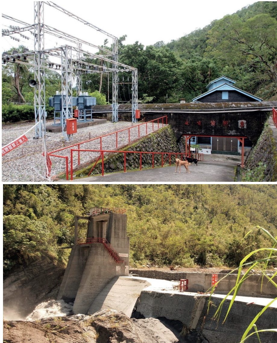
Figure 3.3: The Dongxing Hydroelectric Power Station (originally called the Tanan Power Station) is situated on a branch of the Rijia River, with its water inlet pictured below. The dam, enlarged when Taipower raised the dam wall based on Japanese design, was regarded by local actors as a cause of the degradation of the river's aquatic ecosystem along with several weirs constructed by the semi-official irrigation association and the state-run water corporation for the Taitung area. The relentless generation of cheap energy and cheap water through appropriation of the river's potential for the Taromak symbolized the encroachment of state power on the tribe along with the processes of colonization and modernization, thus becoming central to their campaign for tribal autonomy. Source: Photos taken by the author.
