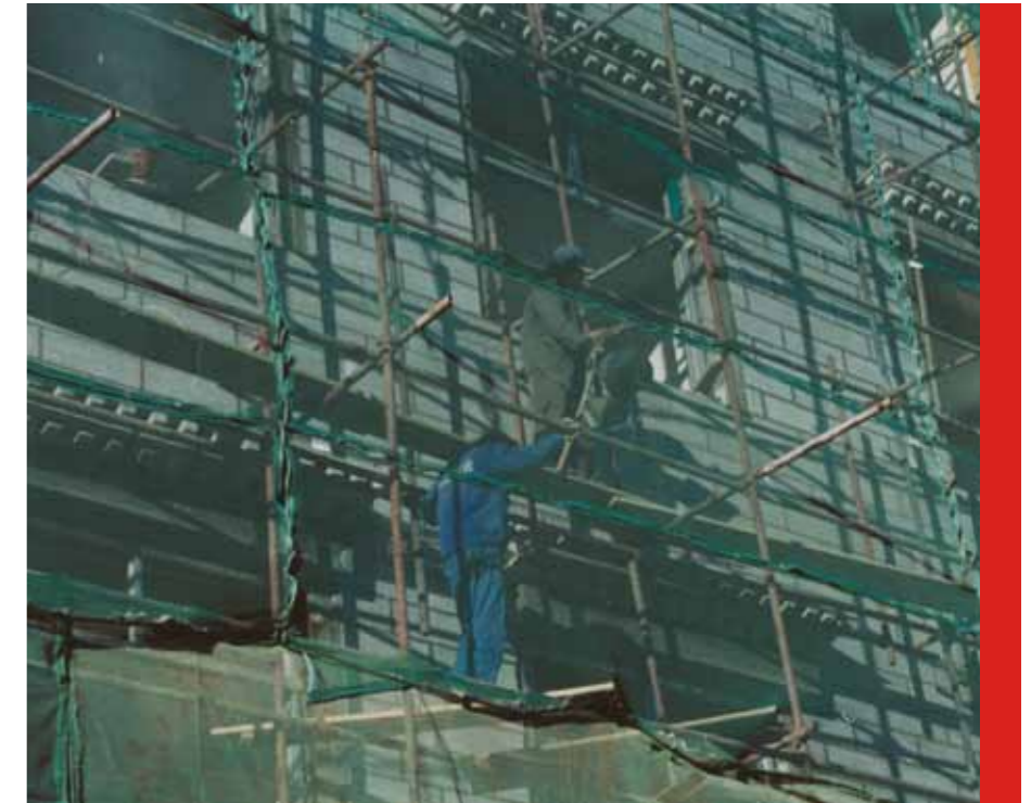
An urban construction site / Andrew Fischer
