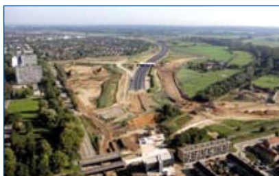
Figure 4.2: Tunnel Roermond, North side entrance ( www.vialimburg.nl ).
