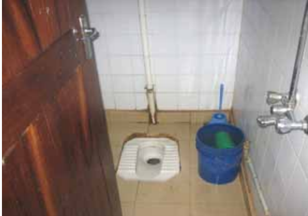
Picture 5: Toilet Facility, Private Dispensary, Non-Squatter Area
