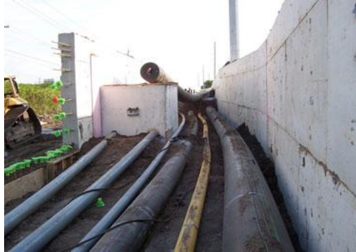
Figure 6.2 Structure to house the utility facilities for 12 companies
