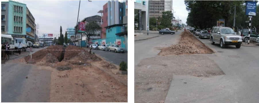
Figure 4.13 Road section cut for underground sewer along Bagamoyo Road
