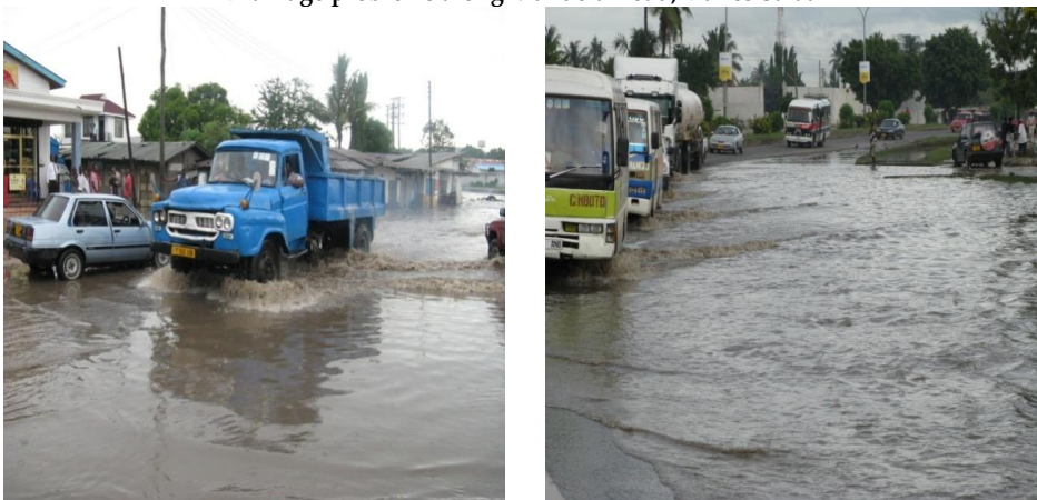
Figure 4.4 Drainage problems along Mandela Road, Dar es Salaam
