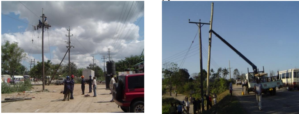
Figure 4.10 Relocation of electricity poles and cables
