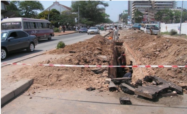
Figure 5.24 Excavations within roadway for repair of underground sewer pipes.
