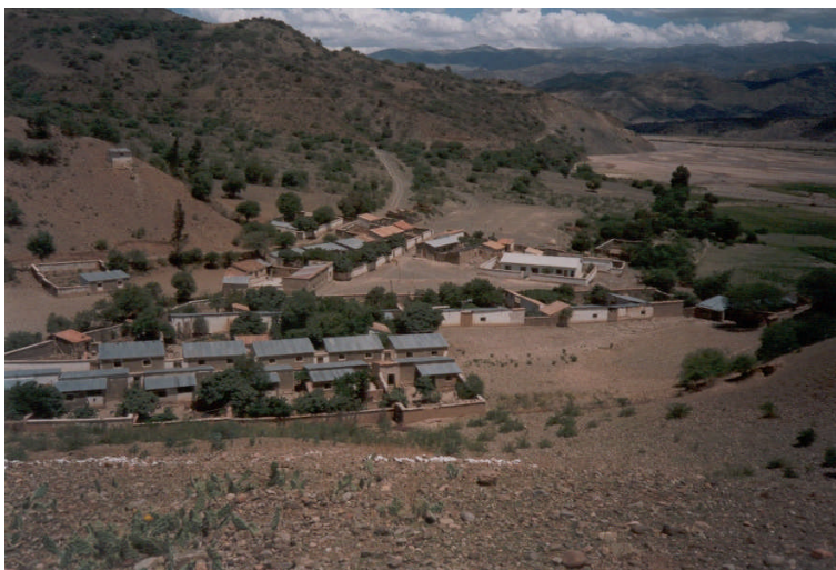
Tuero Chico, the concentrated settlement along the Pilcomayo river (1996) Source: PIED Andino, Miriam Vargas.
