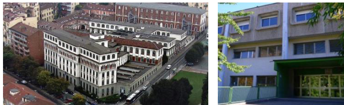
Figure 1. A. Avogadro (school A, left) and J.C. Maxwell (school B, right) Institutes: external views
